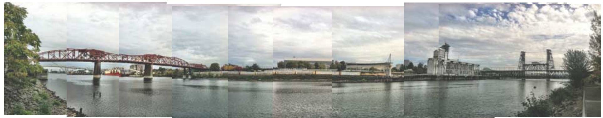
view across willamette to site from base of steel bridge
